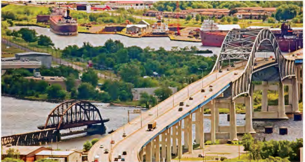
Blatnik Bridge. Photo: Randen Pederson under Creative Commons licensing
